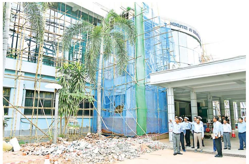
Vice-Senior General Soe Win inspects the renovation works on the office buildings at the Ministry of Electric Power.
