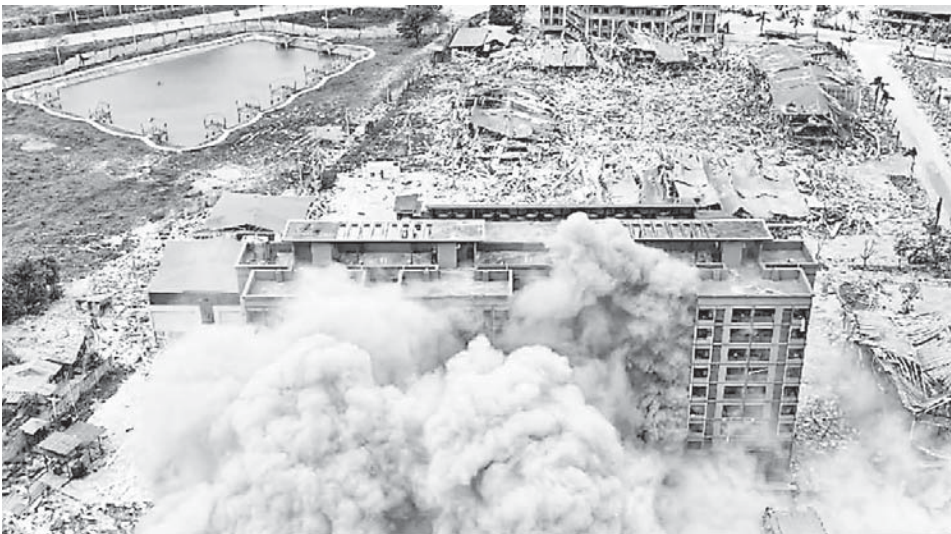
Online scam and gambling buildings being blown up in KK Park.
