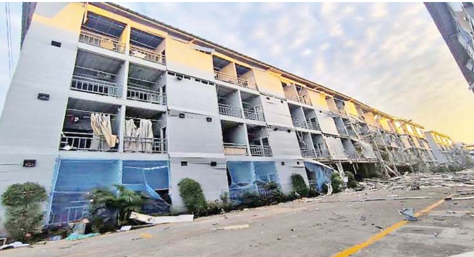
Four storey residential building C9.
