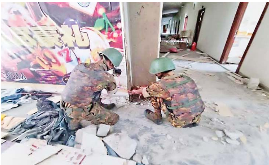
151 kilograms of explosives are used to demolish the four storey residential building C9.
