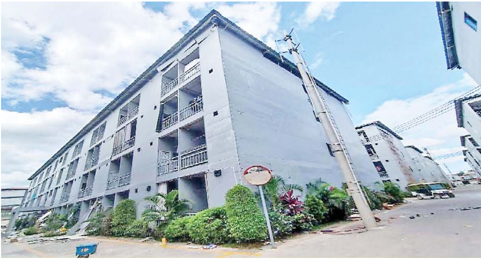
Four storey residential building C12.
