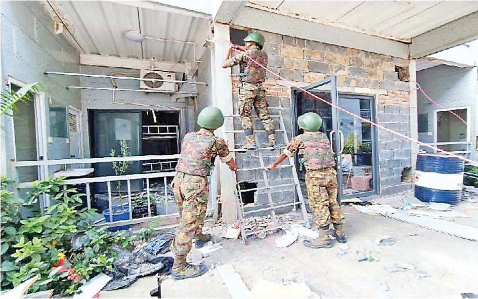
Soldiers installing 151 kilograms of explosives to demolish the four storey residential building C12.
