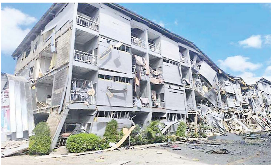
The demolished four storey residential building C12.
