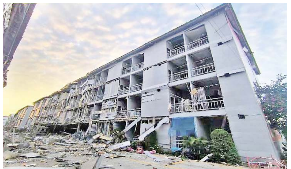
The demolished four storey residential building C9.
