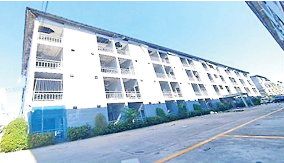
Four-storey residential building C6.
