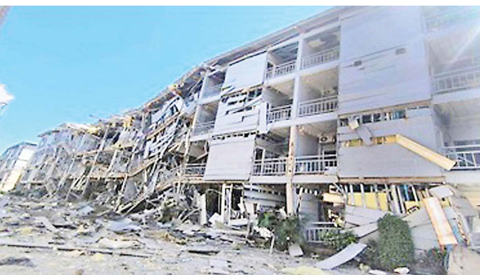
The demolished four-storey residential building C6.
