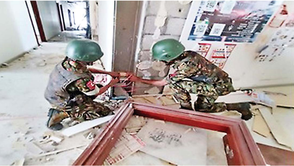
Soldiers installing explosives to demolish the four-storey residential building C6.
