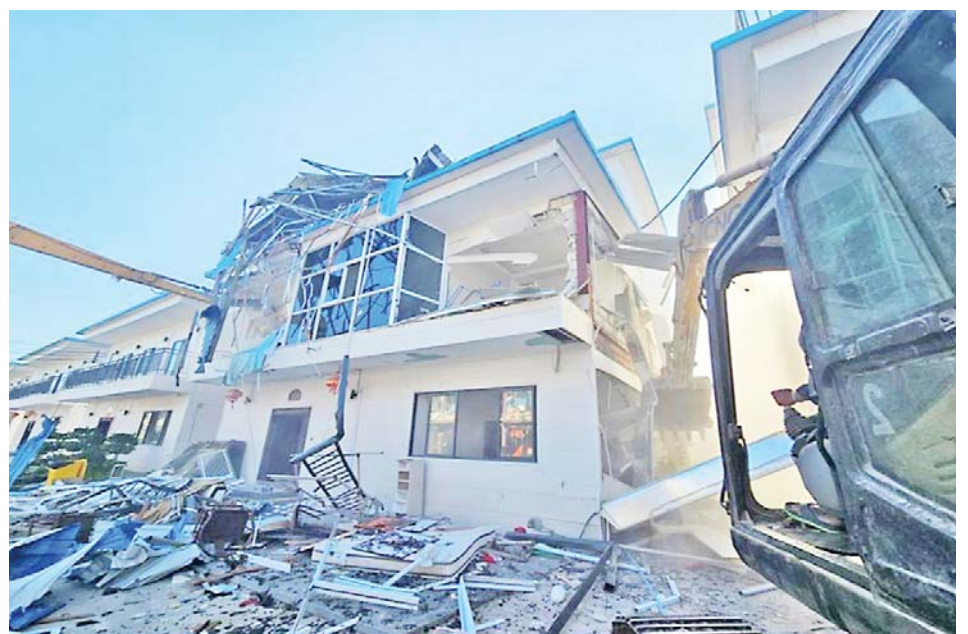
Demolition of buildings used in online scams and gambling in KK Park with the use of heavy machinery.
