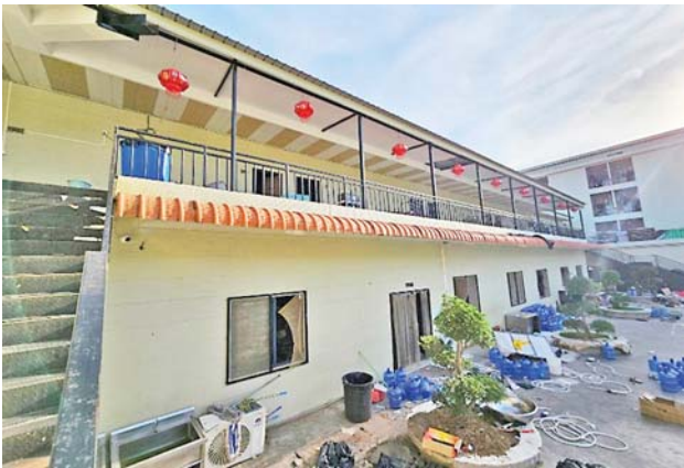
A two-storey building in KK Park that will be destroyed with heavy machinery.
