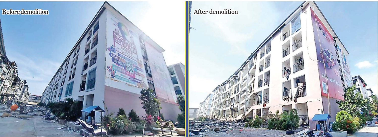
A documentary photograph showing demolished five-storey building C-11, which was illegally built in Part-3 of KK Park.
