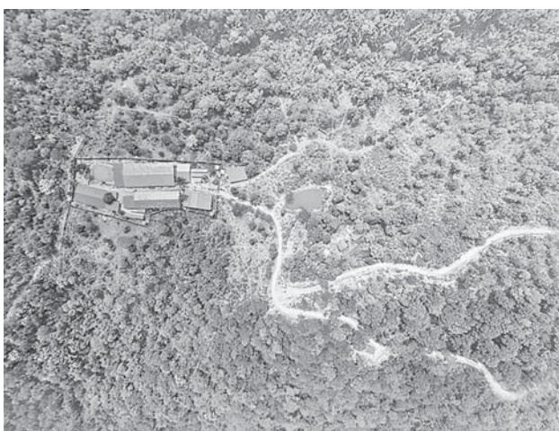
Buildings used in online scam and gambling operations near Panku Village, Tachilek City.
