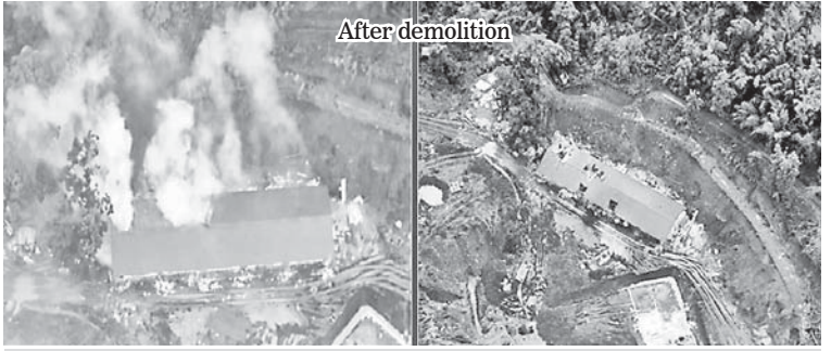
After demolition Permanent demolition by explosives of residential buildings used for online fraud and gambling activities in Myawady Township, Kayin State (13 August 2026).
